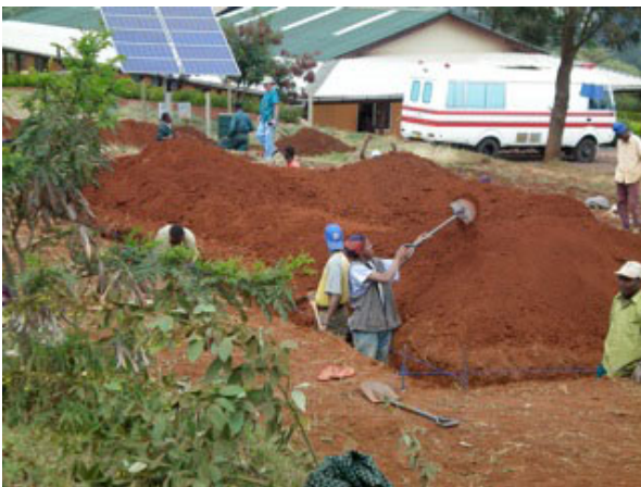
Health Center construction crew at work
